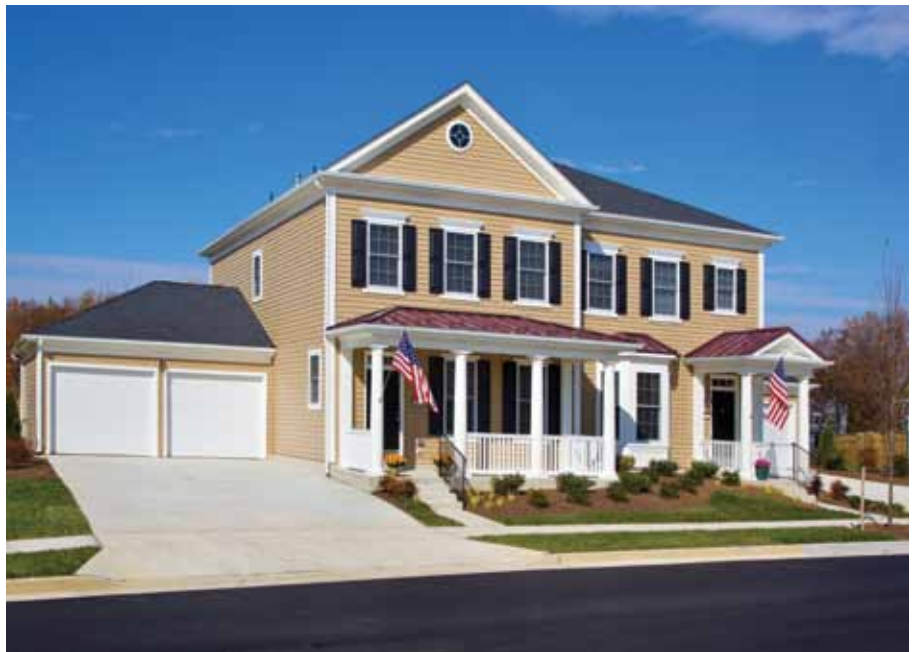
The completion of Liberty Park at Andrews (facing page and above) marks the delivery of 85 out of 415 total new and renovated homes planned for Joint Base Andrews under the AMC East development plan.
